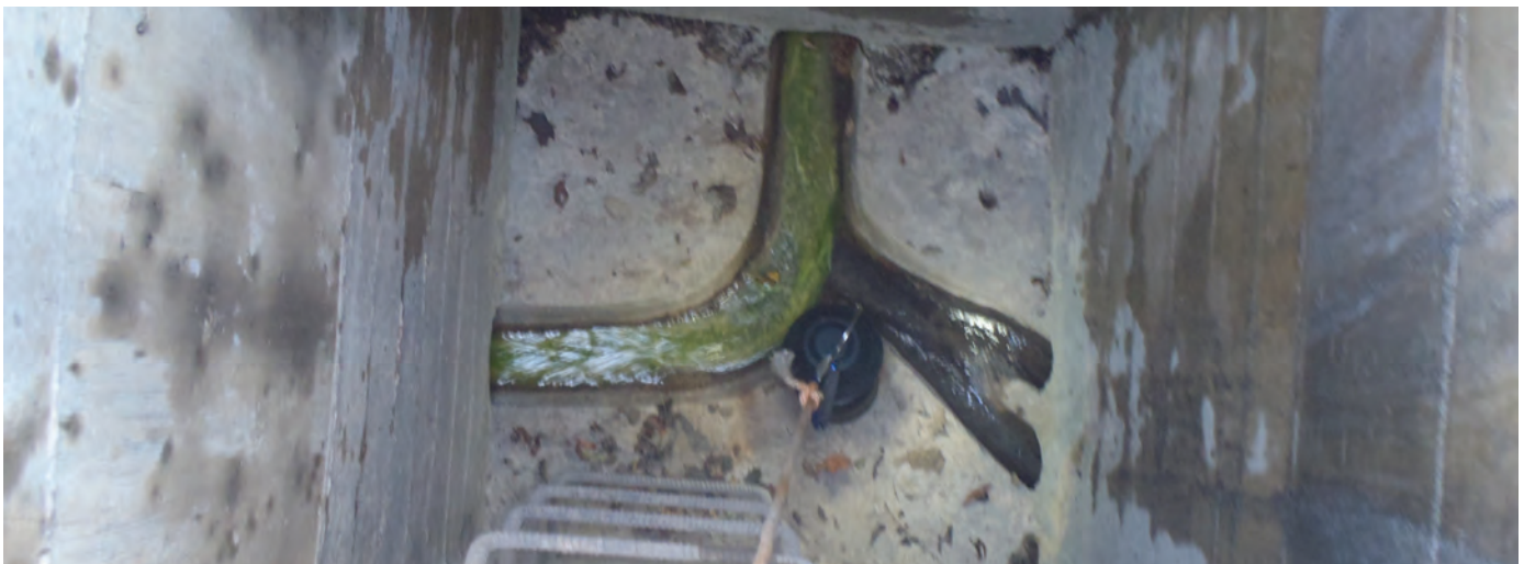
Figure 7 – Dye Testing in the City of Vaughan
