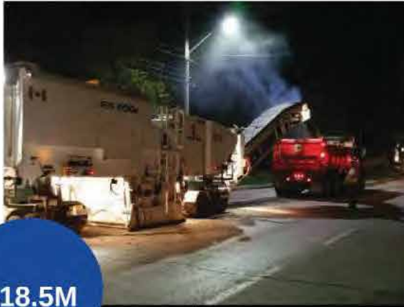
Road Rehabilitation and Preservation
