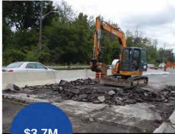
Bridge and Culvert Rehabilitation
