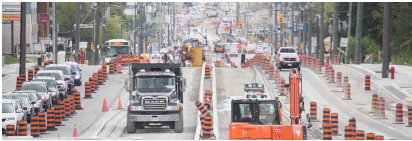
Construction on the Davis Drive rapidway, Town of Newmarket
