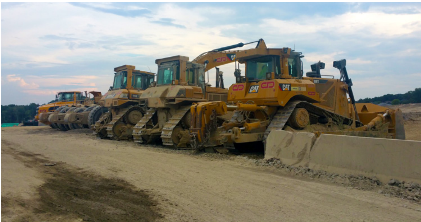
Construction equipment at a residential development, Town of East Gwillimbury
