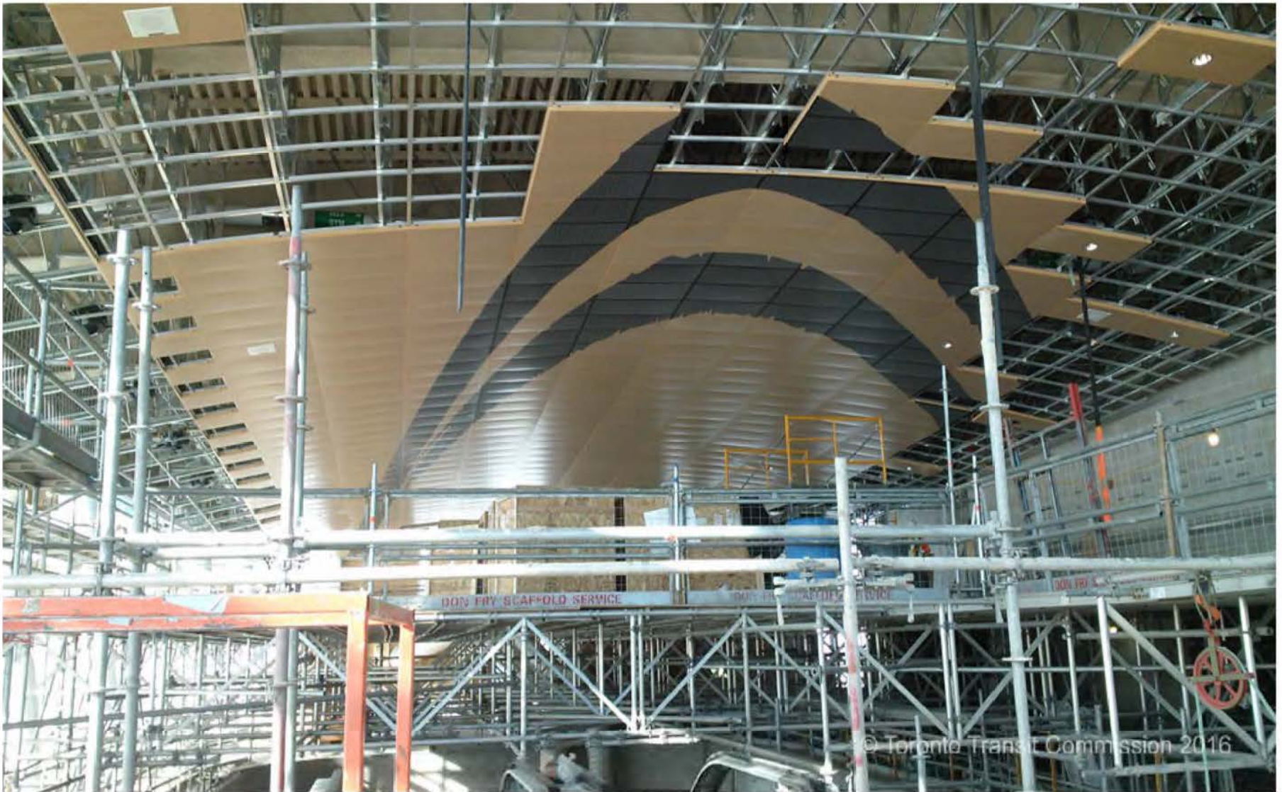
Downsview Park Station East entrance ceiling tile installation with “Spin” artwork
