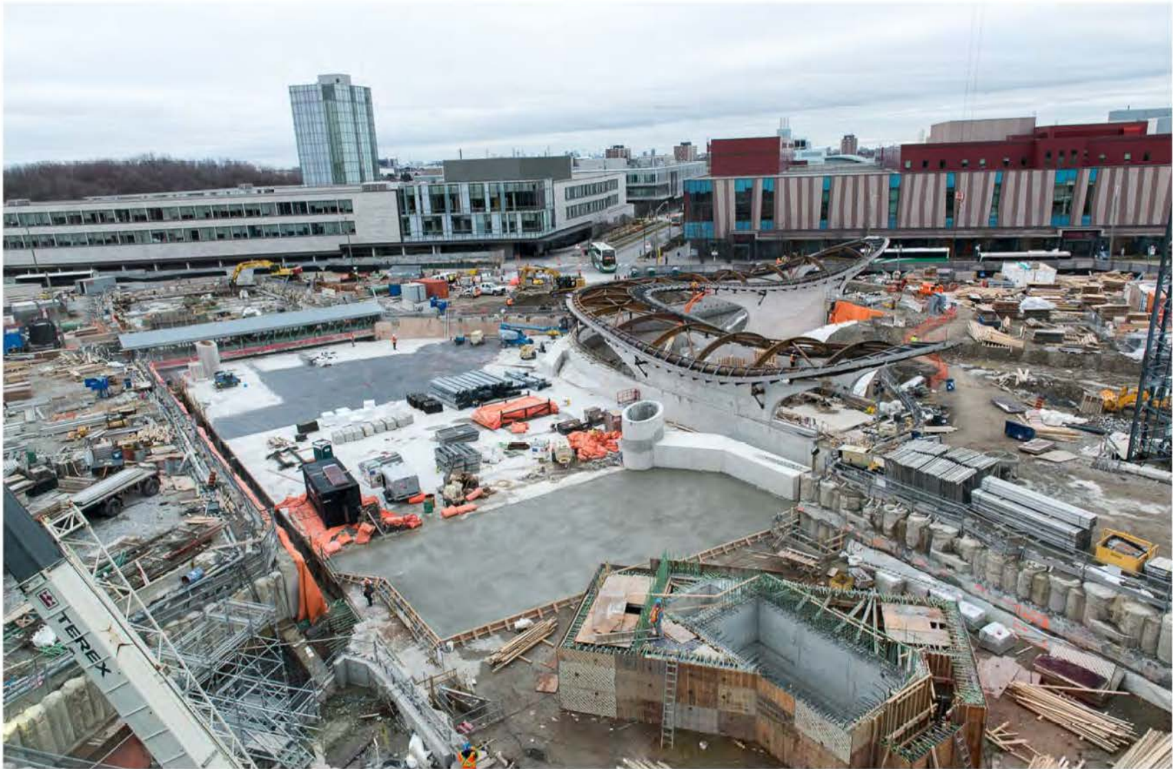
York University Station Station box roof pour complete
