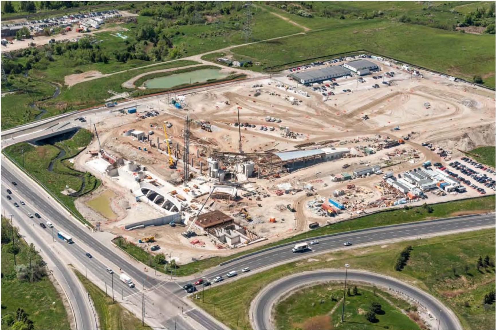
Highway 407 Station Aerial view looking southwest
