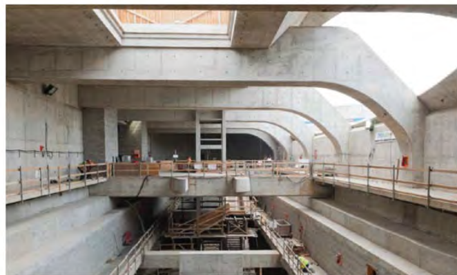
Interior view of the station including the skylight. – May 27, 2015
