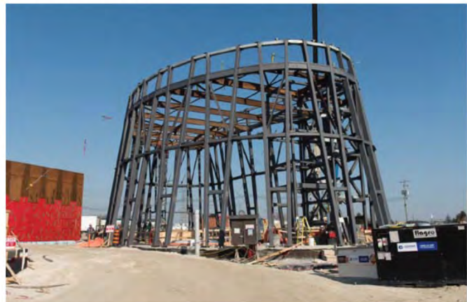
Station entrance and power substation (on left). – December 14, 2015
