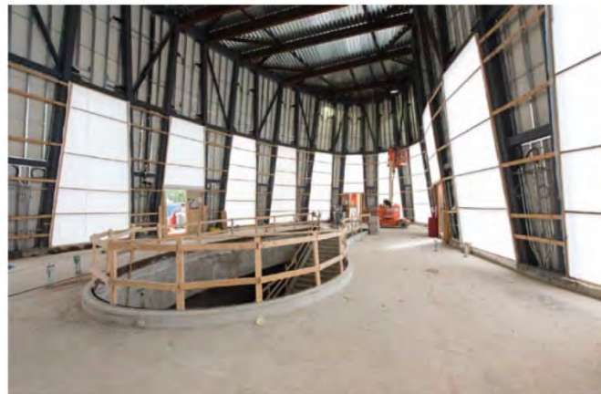
Station entrance (interior view). – December 14, 2015
