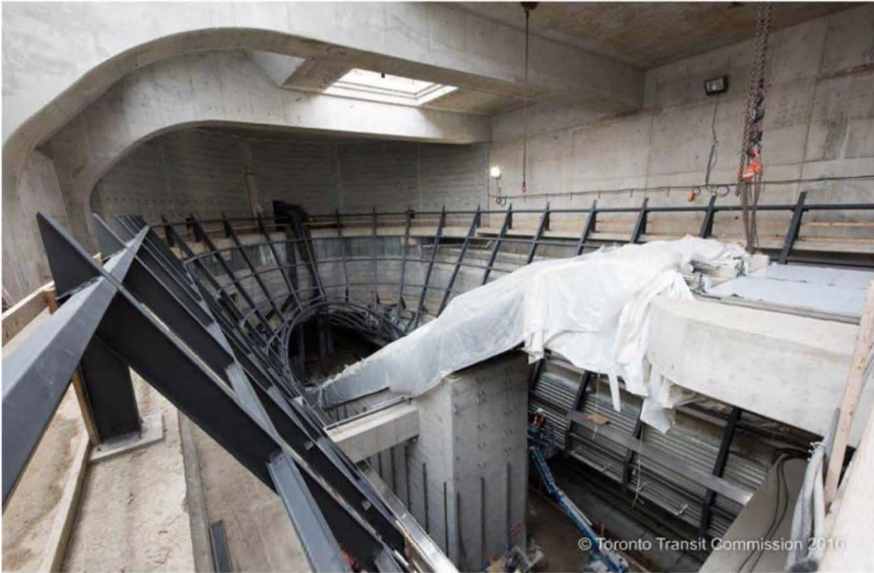
Highway 407 Station South escalator from concourse to platform installed
