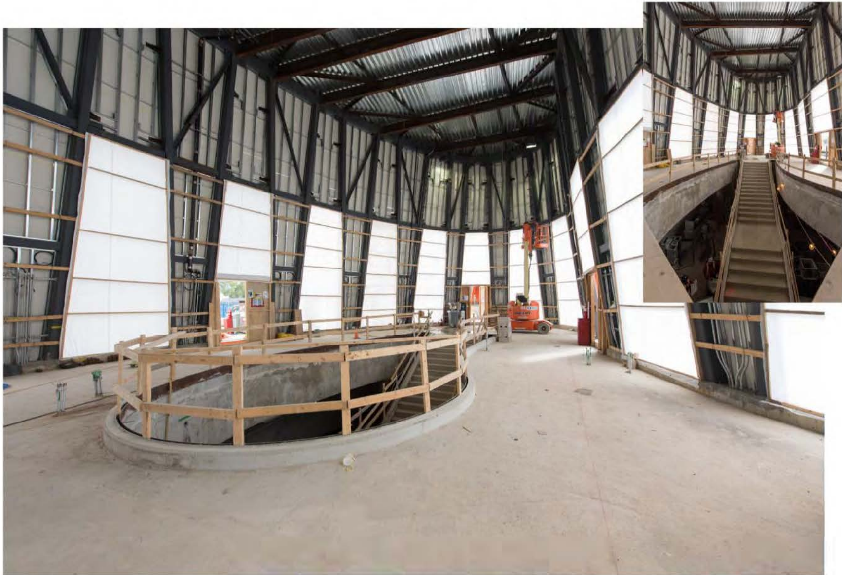
Pioneer Village Station Interior of the south entrance
