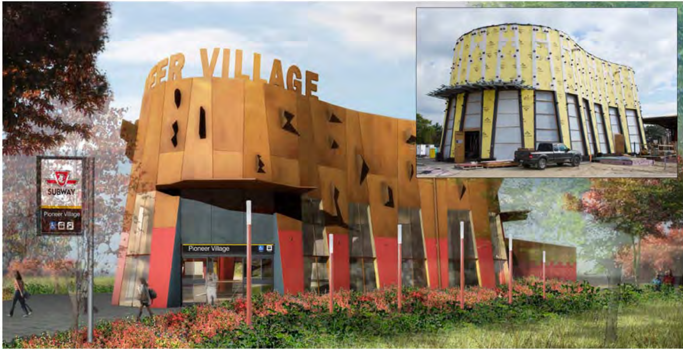
Above: Station south entrance rendering. Inset: Entrance progress. – December 14, 2015
