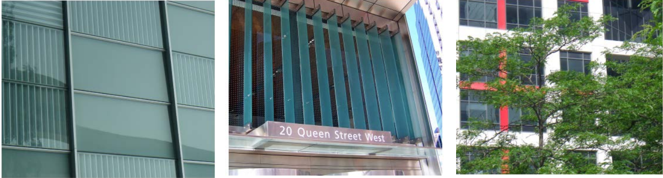
Pictures showing internal blinds, external coverings, and mullions Source: Markham Bird-Friendly Design Guidelines
