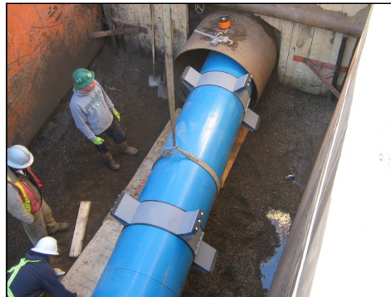
Jack & Bore Construction Method
