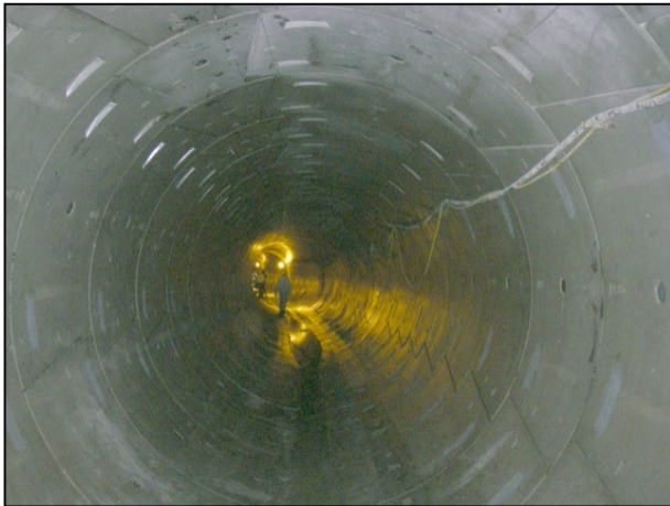
Segmental Lining Tunnel
