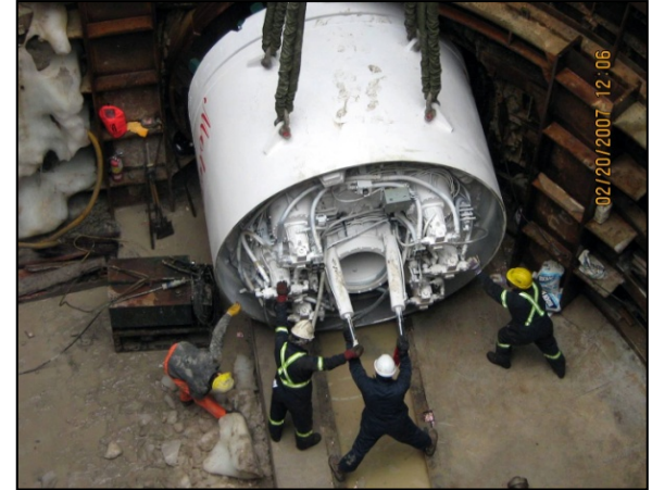
Tunnel Boring Machine
