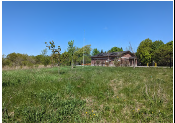
PHOTO 8: View of the southern portion of the Site, facing northwest.
