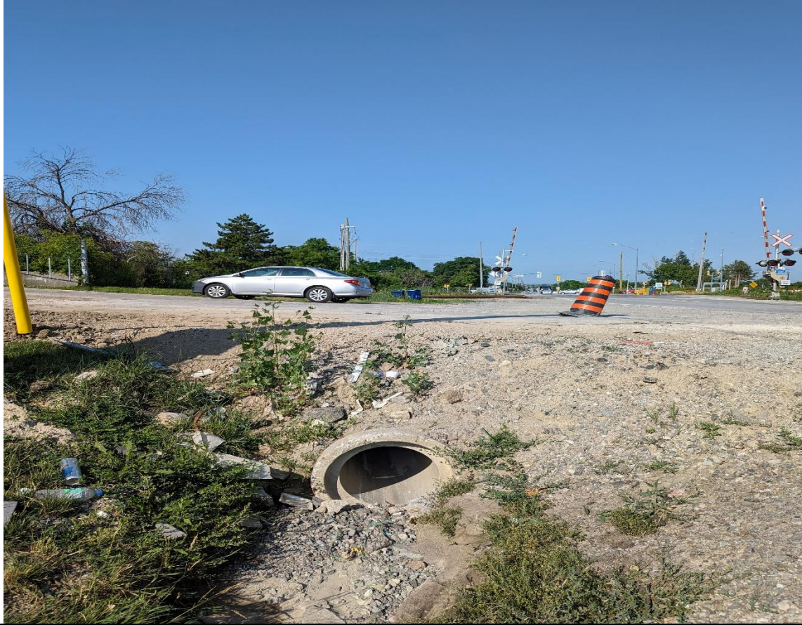
Site Photograph Photo of Culvert "Rail South"
