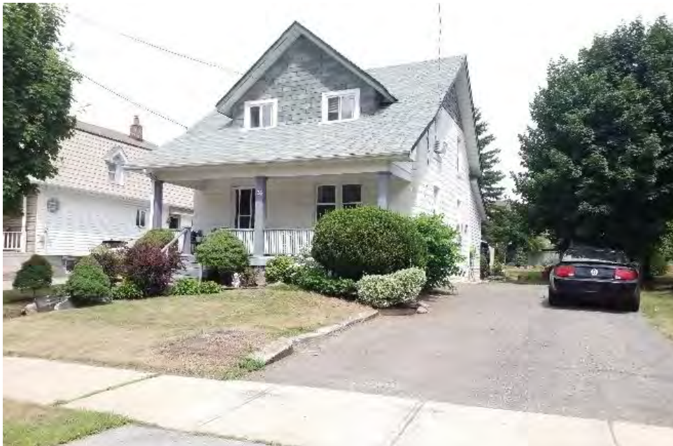
Looking northwest towards the residence at 24 Railway Street.
