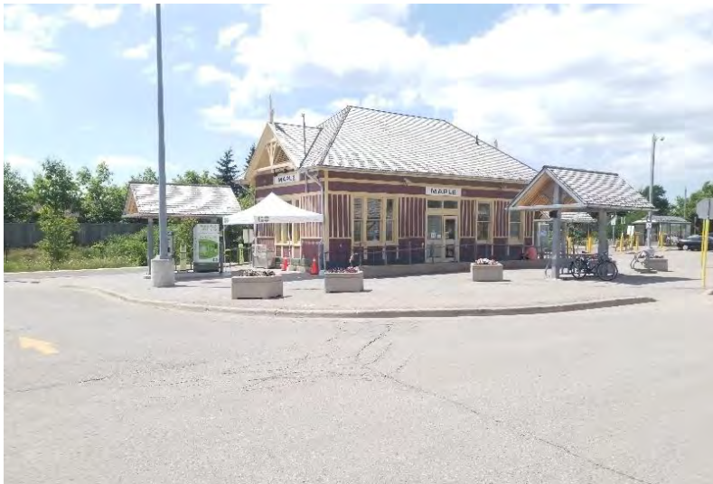
Looking northwest towards the Maple GO Station.
