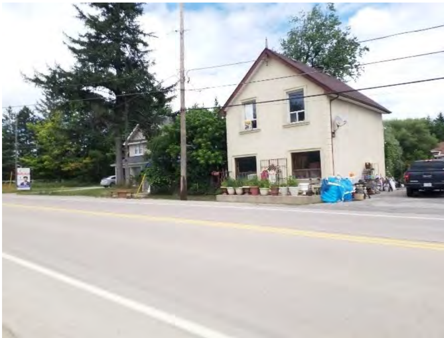
Looking northeast towards the residence at 10953 Jane Street.
