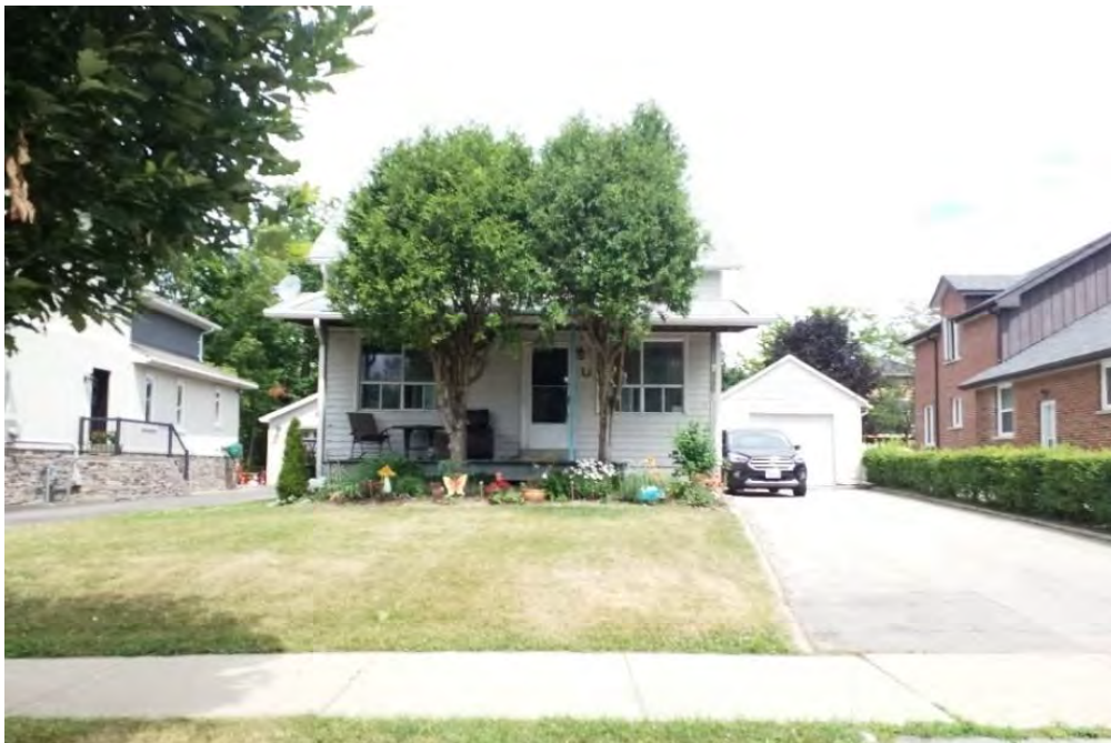
Looking north towards the residence at 14 Railway Street.
