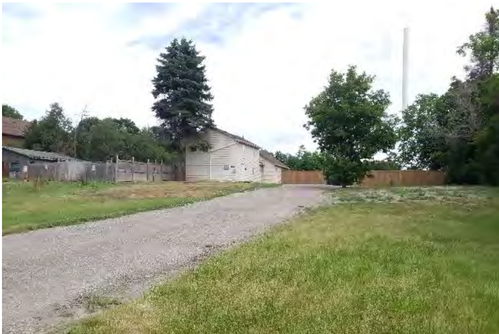
Looking northeast towards the residence at 10811 Jane Street.
