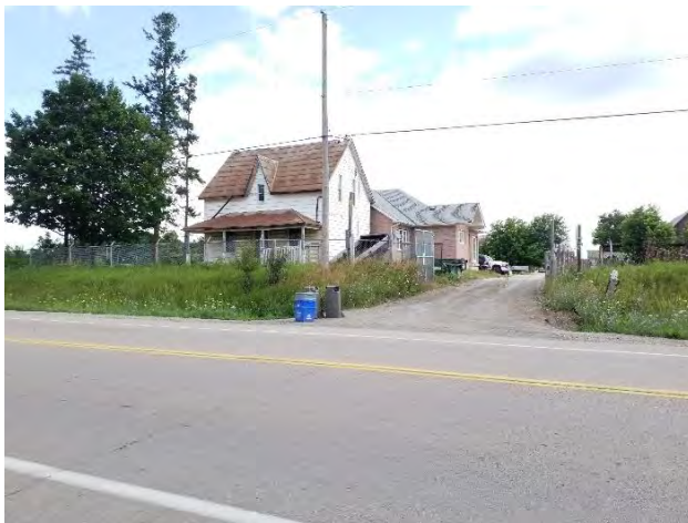
Looking northeast towards the residence at 11451 Jane Street.
