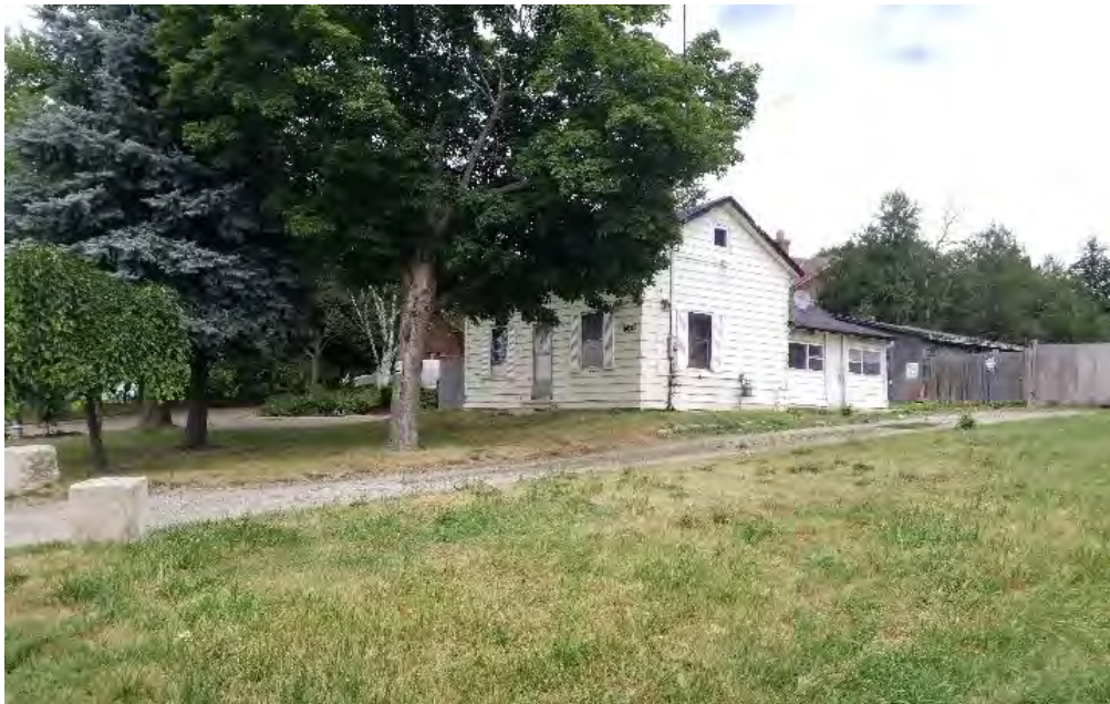
Looking north towards the residence at 10819 Jane Street.
