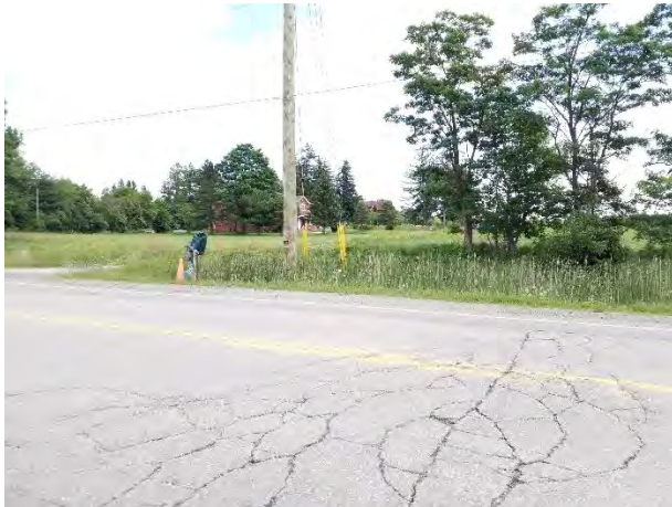
Looking northeast towards the property at 11151 Weston Road.
