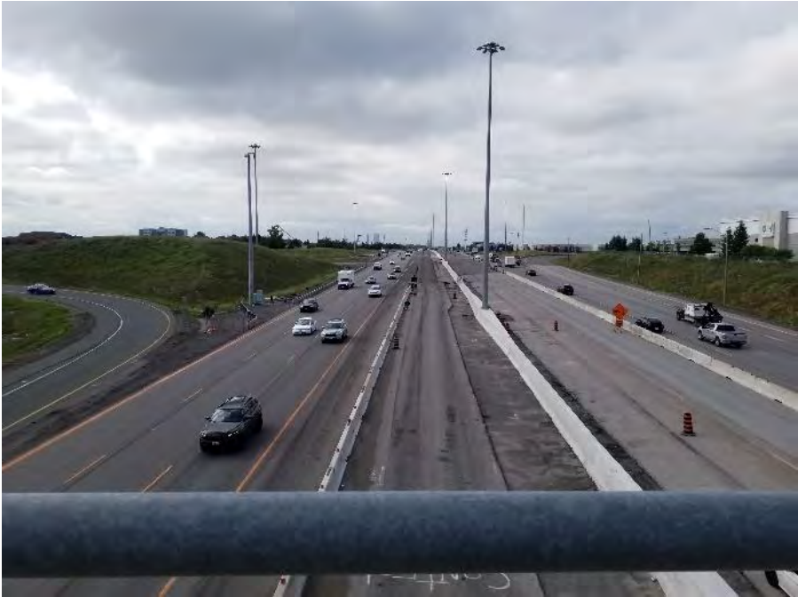
Plate 3: Highway 400, looking south from Teston Road near the western limit of the study area.
