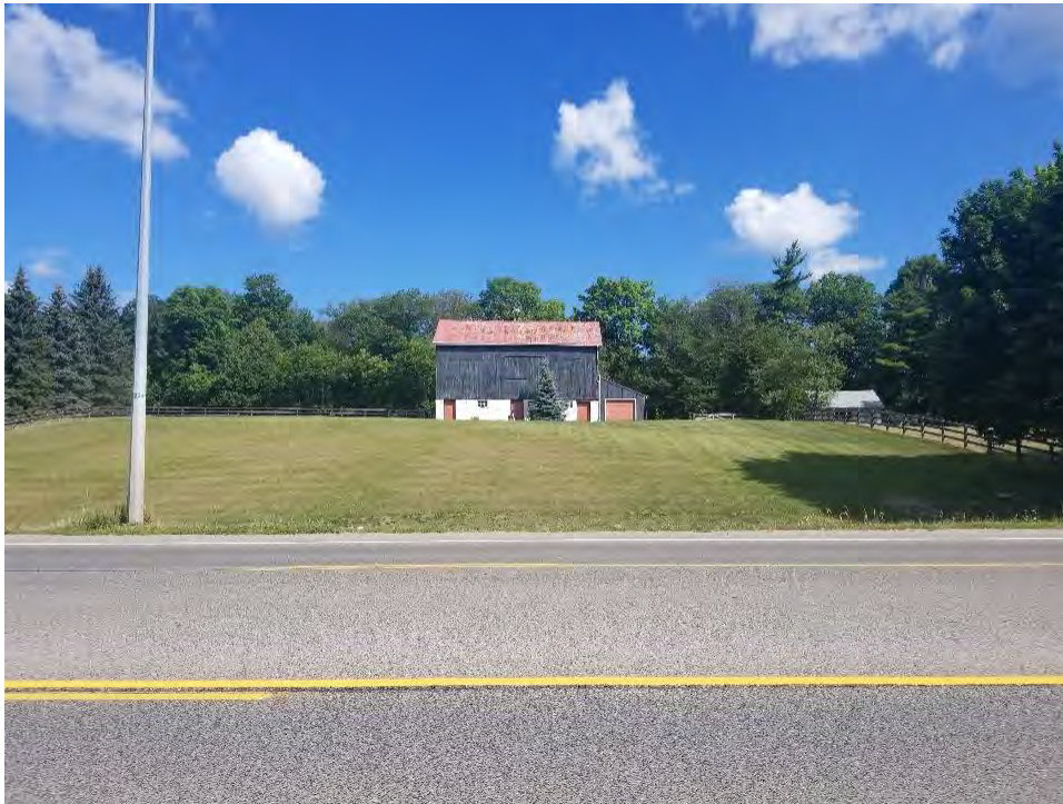
Looking north towards the barn at 1138 Teston Road.
