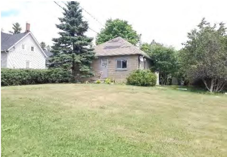
Looking northeast towards the residence at 10885 Jane Street
