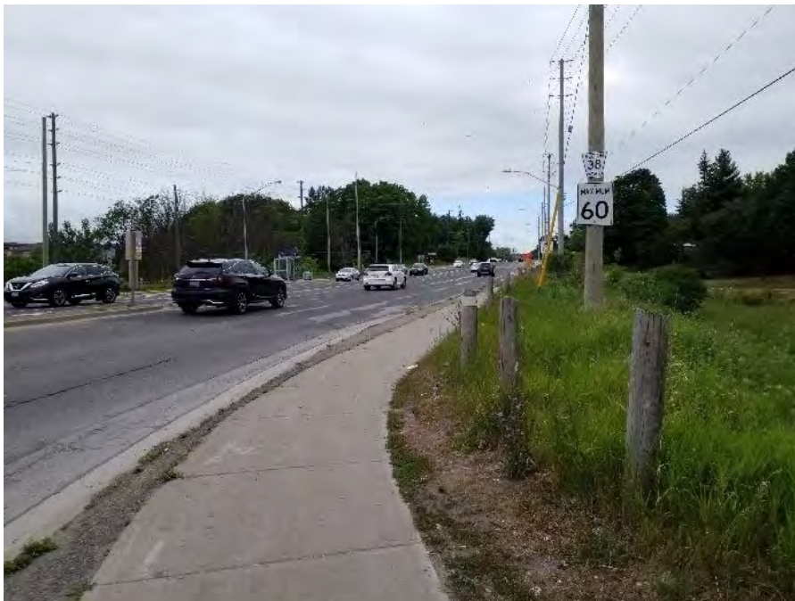
Plate 1: Bathurst Street, looking north from its intersection with Major Mackenzie Drive West near the eastern limit of the study area.
