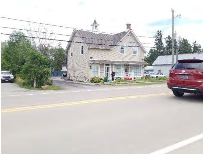
Looking southeast towards the commercial building at 10933 Jane Street.
