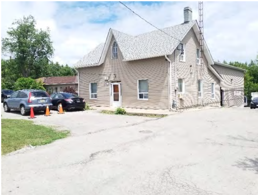
Looking northeast towards the residence at 10945 Jane Street
