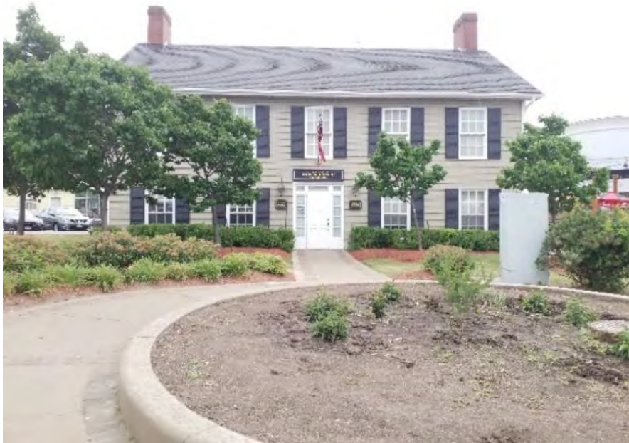
Looking southeast towards the former residence at 2963 Major Mackenzie Drive West.
