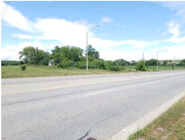
Looking northeast towards the former residence at 2546 Teston Road.
