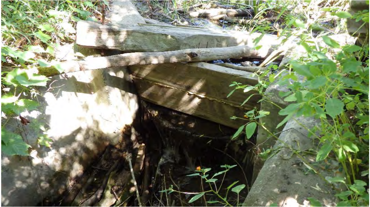
Photo 1: Fisheries Site 1 - Dam outfall and fish passage barrier at upstream edge of survey area
