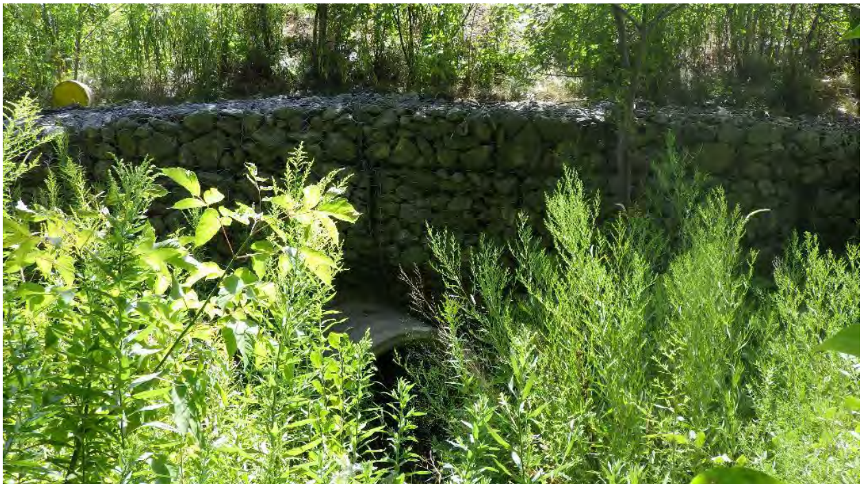
Photo 16: Fisheries Site 3 - Culvert inlet and headwall upstream of Teston Road
