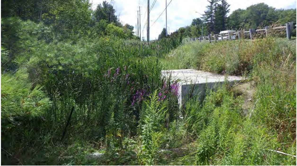
Photo 11: Fisheries Site 2 - Culvert outlet downstream of Teston Road
