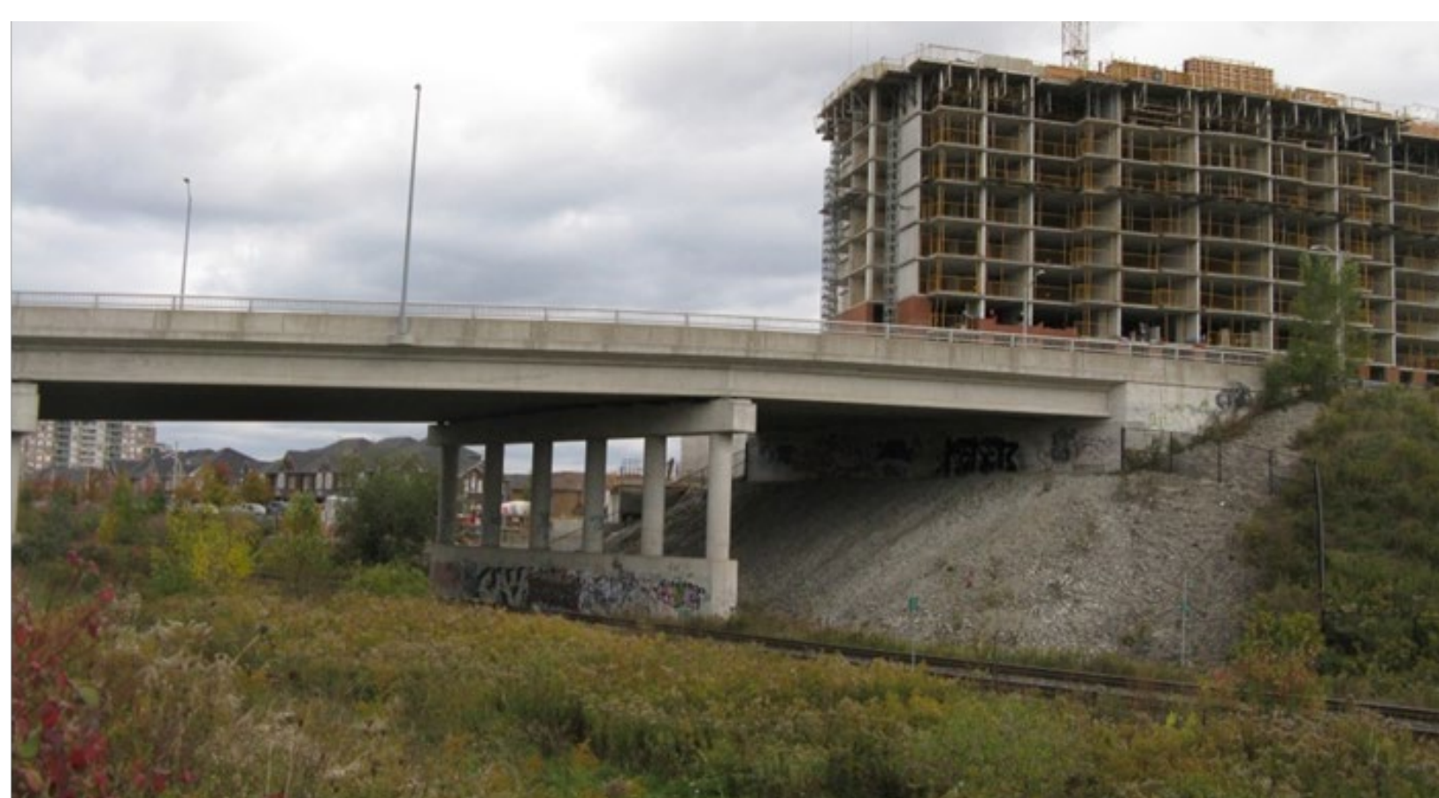
Overpass example: Bantry Road east of Yonge Street.
