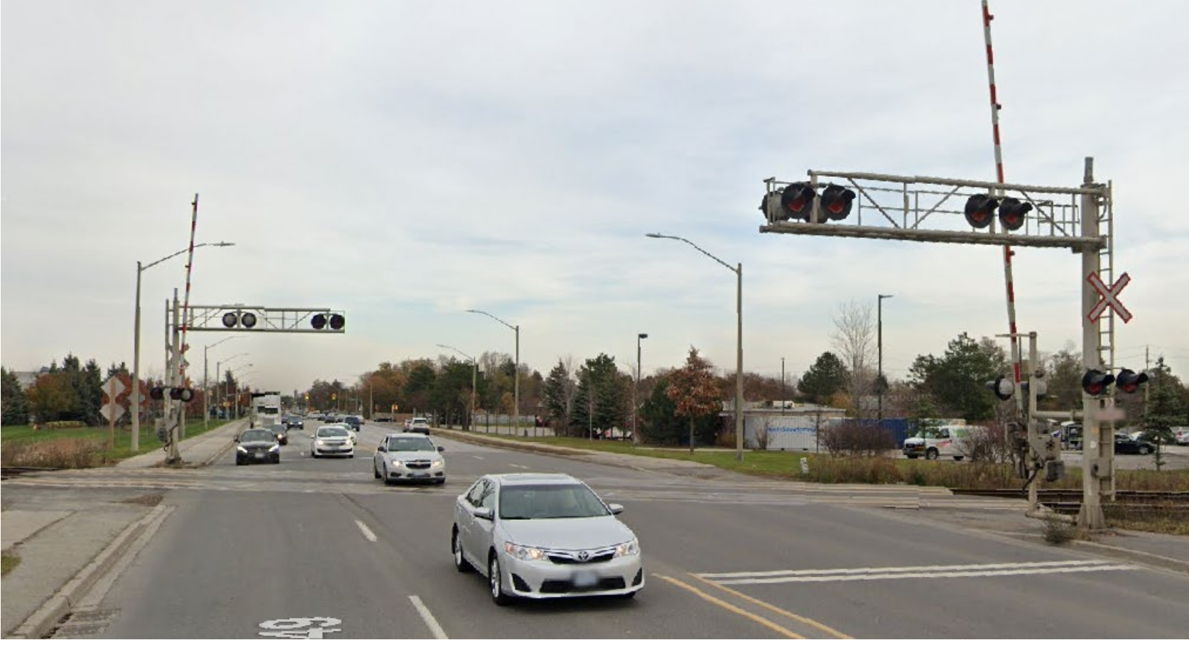
Existing Elgin Mills Road at-grade crossing East of Yonge Street.
