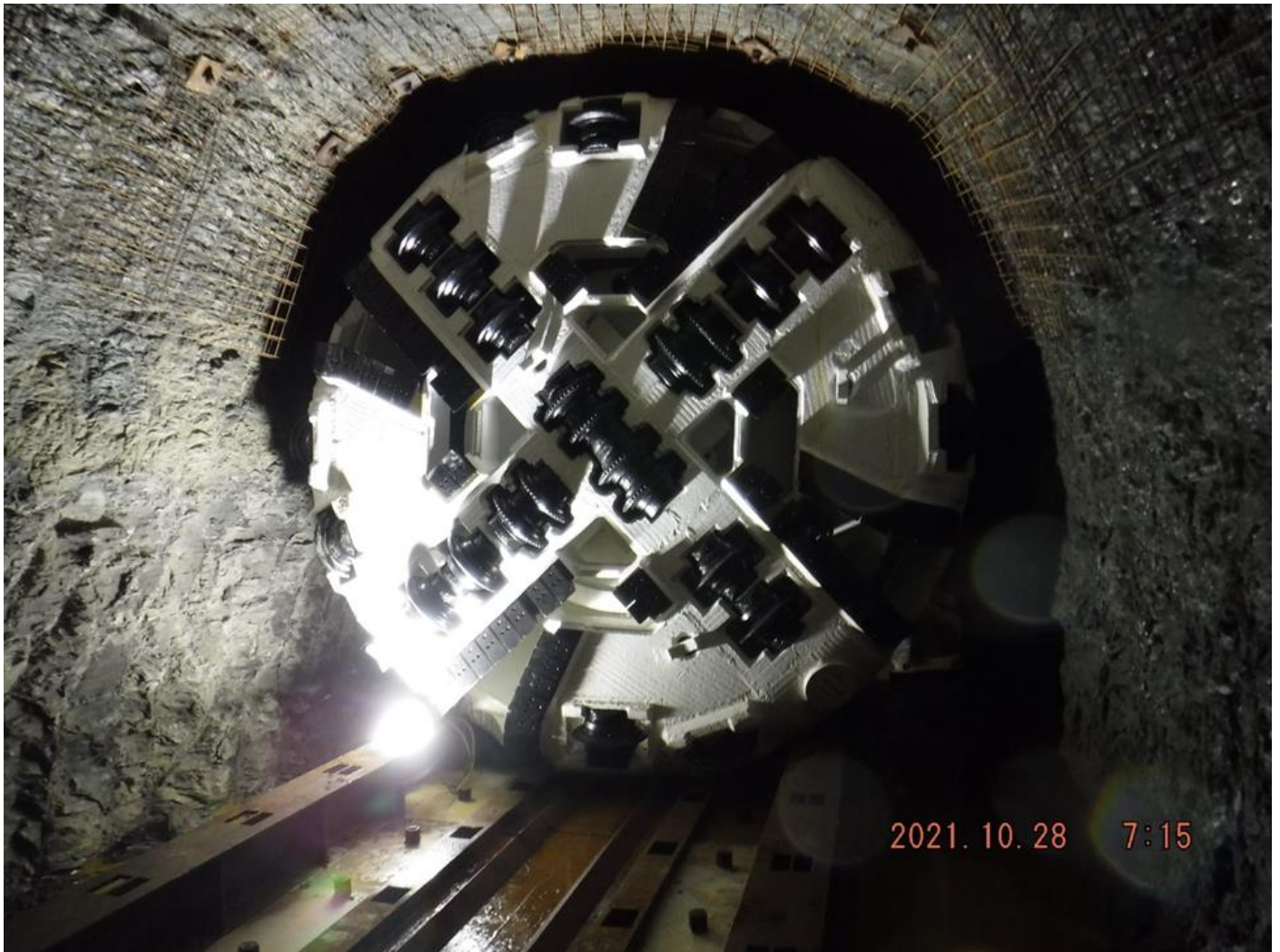
Figure 10.19 Photo of Rock TBM Facing Cutterhead
