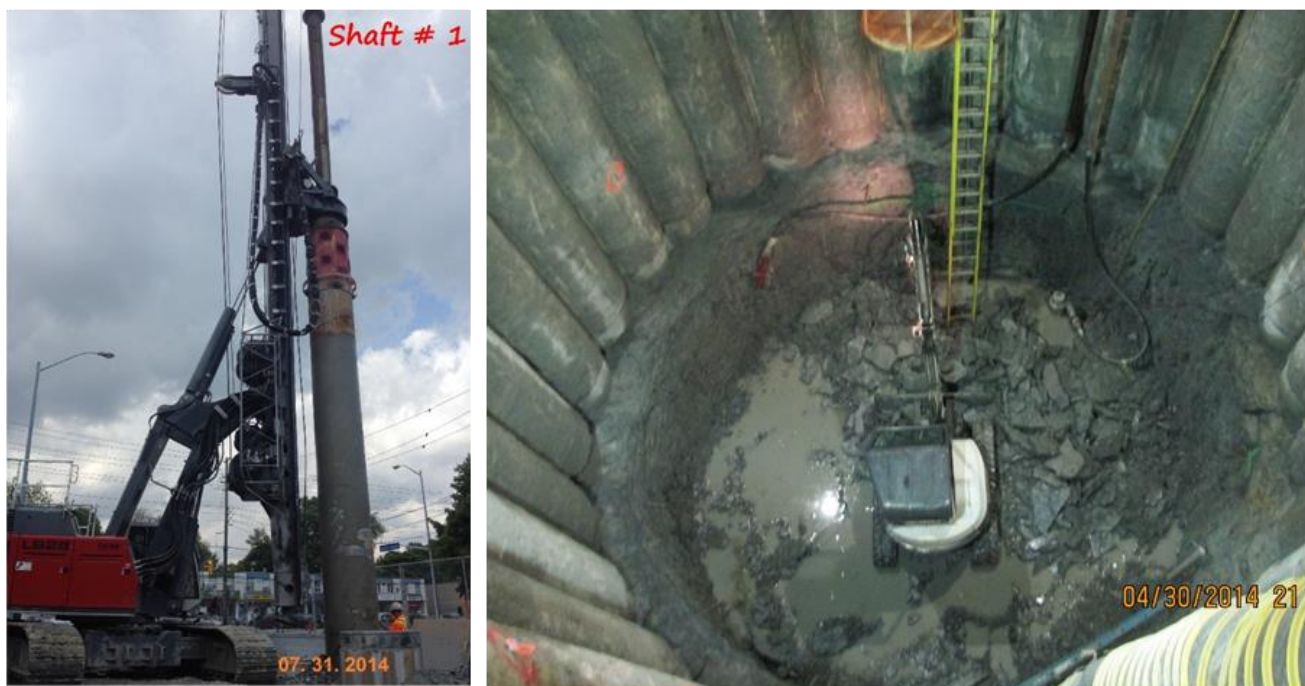
Figure 10.16 Secant Pile Drill Rig (left) and Installed Secant Piles (right)
