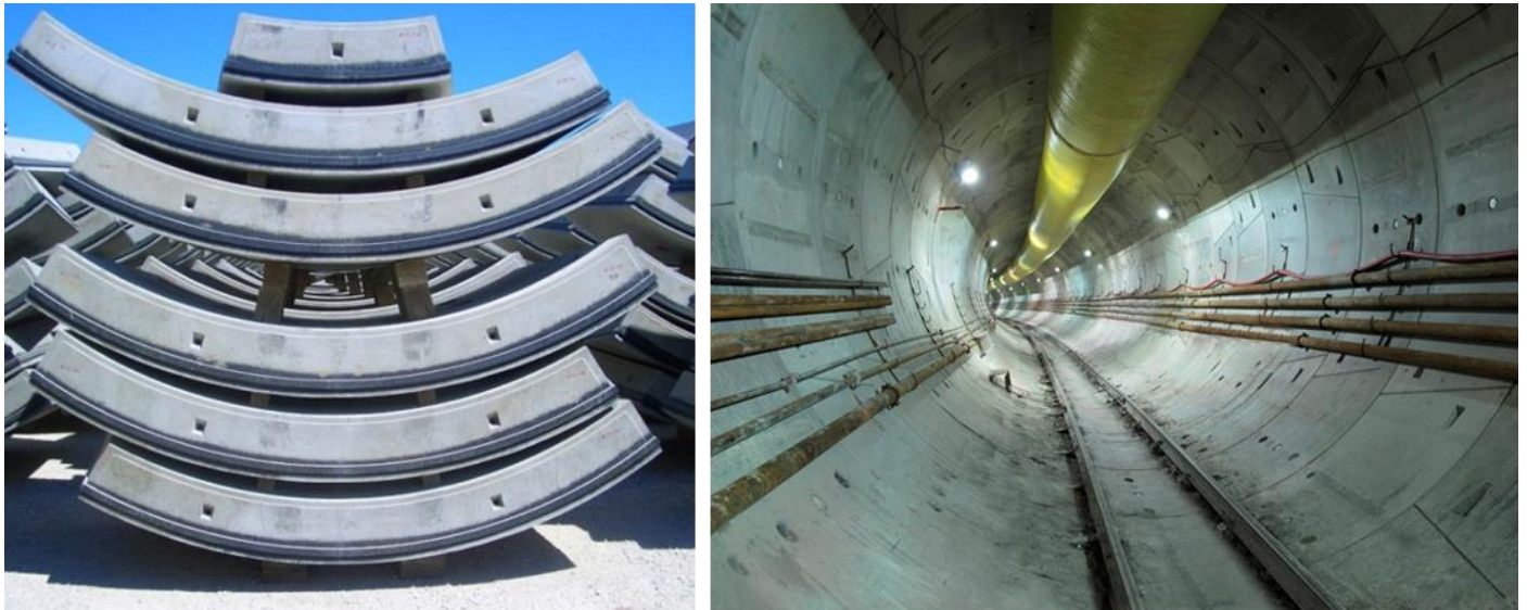
Figure 10.21 Precast Concrete Tunnel Lining
