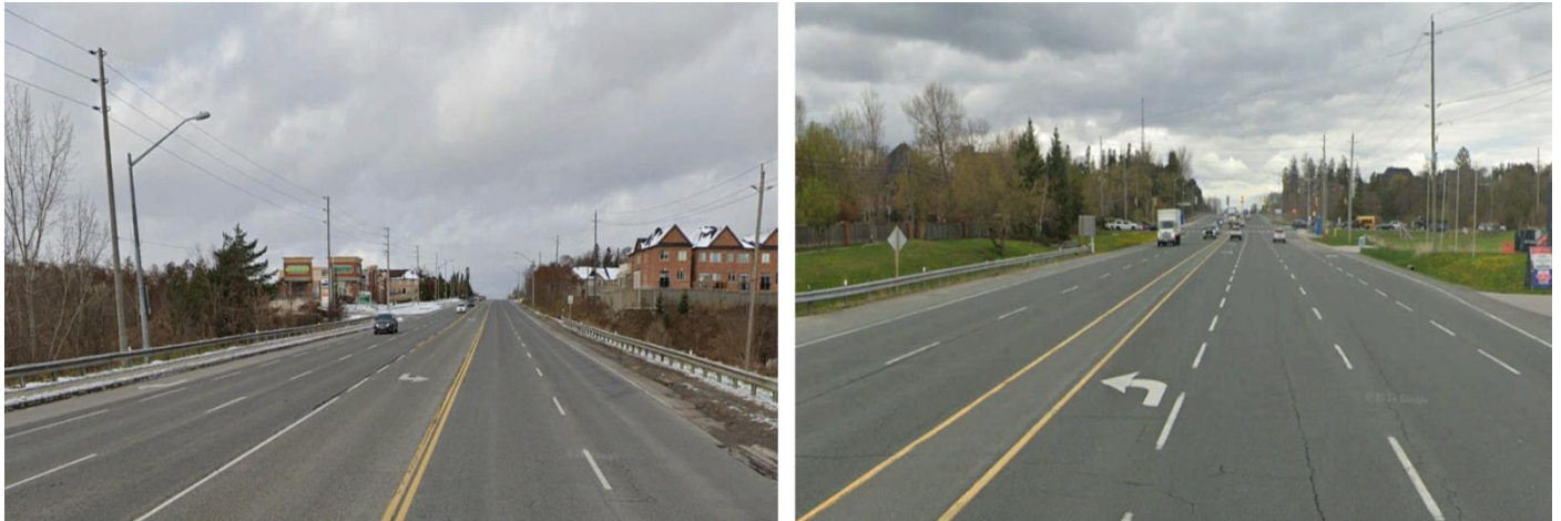
Figure 6.19 Yonge Street Looking north (1) from Jefferson Forest Drive, (2) Toward Bloomington Avenue Intersection. (Google Maps "Streetview," digital images http://maps.google.com )
