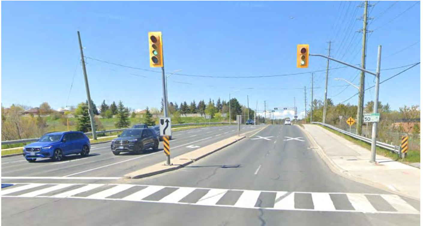
Figure 5.17 St. John's Sideroad Looking West Towards the Rail Crossing West of Industrial Parkway. (Google Maps "Streetview," digital images http://maps.google.com )
