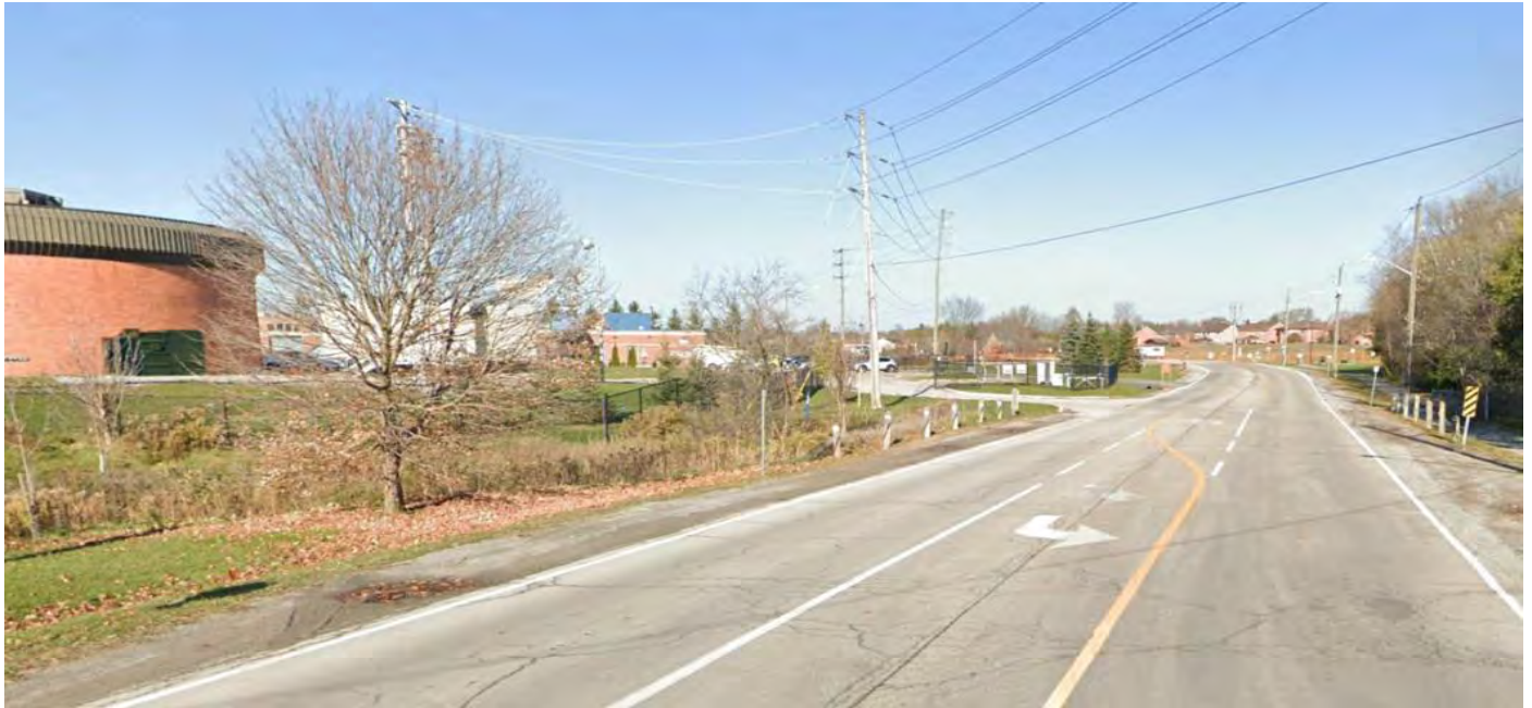
Figure 5.8 Bayview Parkway Looking North Towards the Existing Newmarket SPS (Google Maps "Streetview," digital images http://maps.google.com )
