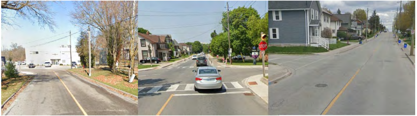
Figure 5.11 (1) Pine Street Looking North Towards Bogart Creek SPS, (2) Prospect Avenue Looking North at Timothy Street Intersection, (3) Gorham Street Looking East at Pine Street intersection. (Google Maps "Streetview," digital images http://maps.google.com )
