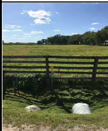
Watercourse Looking Upstream
