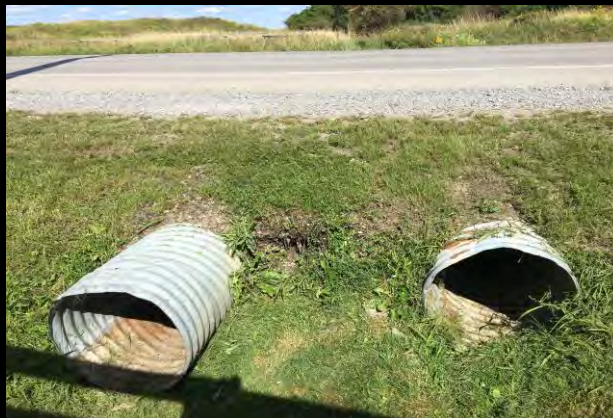
Upstream Structure Face
