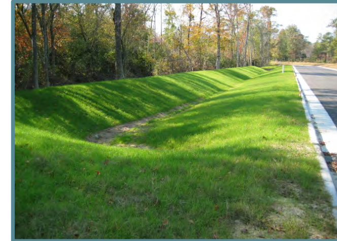
Enhanced grass swales can be applied in road rights-of-ways or along parking lots. Source: Thomas Engineering PA
