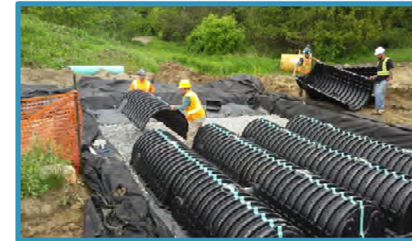
Infiltration chambers being installed. Chamber systems can be large, both in depth and footprint.
