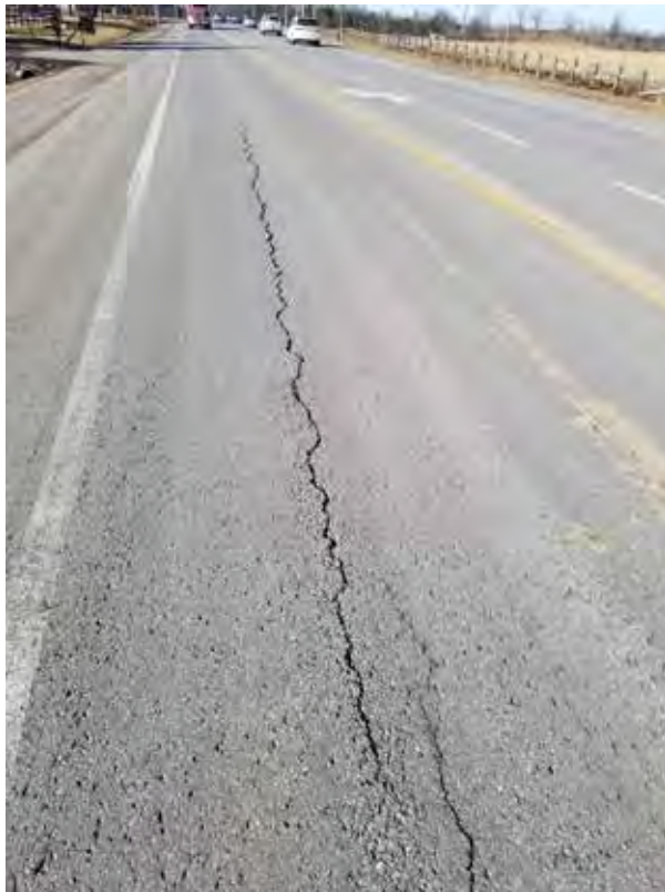
Warden Avenue SB lane, south of intersection with Elgin Mills Road
